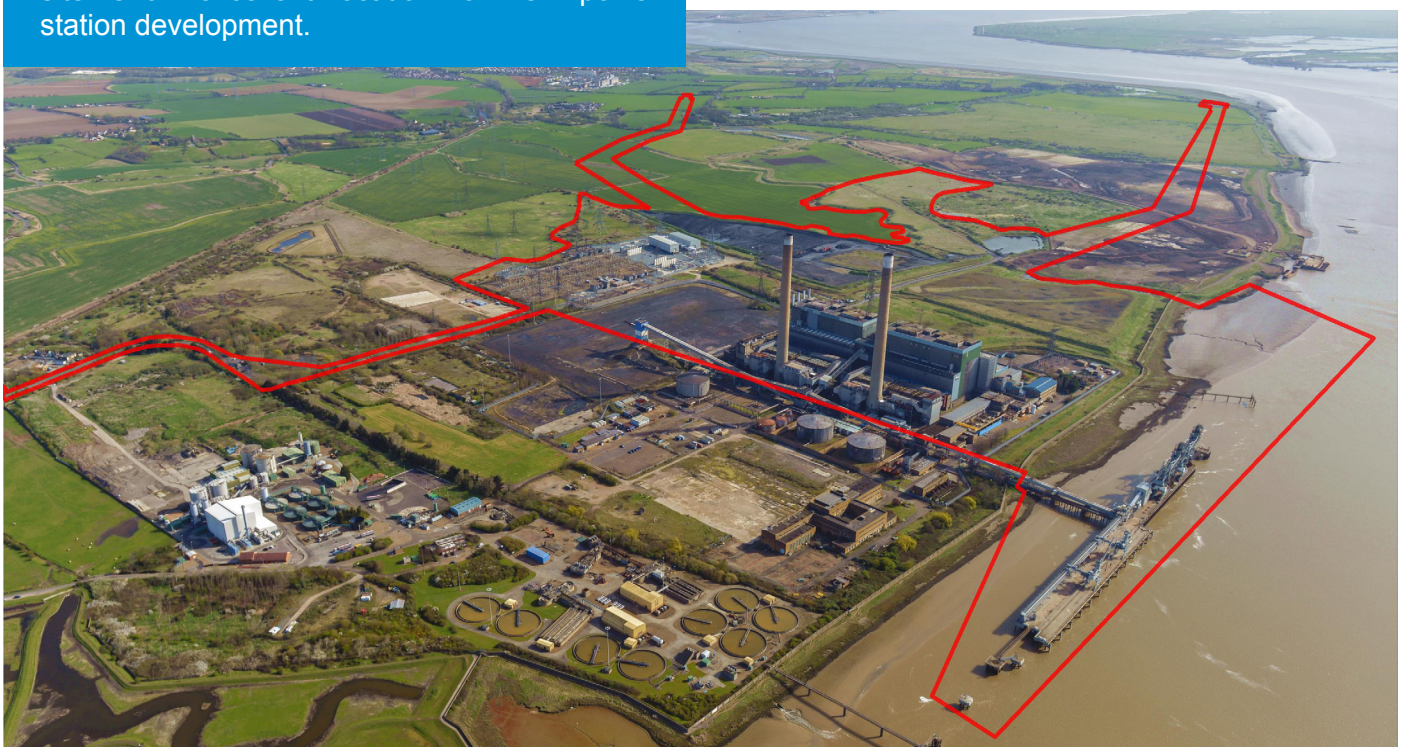
Aerial view of Tilbury B with Tilbury Energy Centre order limits
